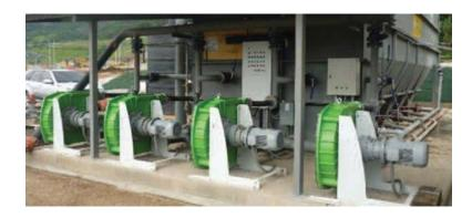
Peristaltic pump hose life is affected by 3 areas: Pump Conditions, Quality of the Hose, and Material Moving Through the Hose.
